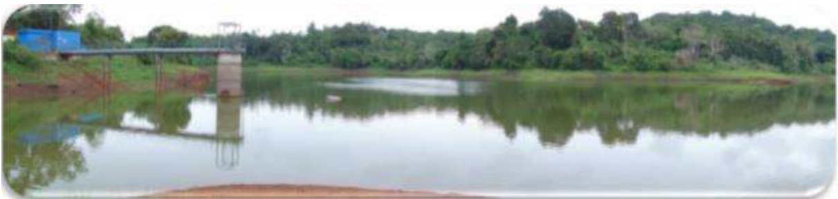
Figure 2- Retenue collinaire de Comani. Source: ARS, 2018.
