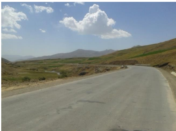
The newly tarred Behsud road
